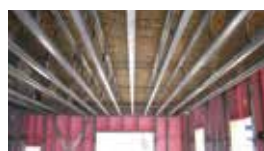
OSB and plywood to iSPAN joists
