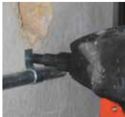
12HSMPO34 clip assembly used to secure conduit
