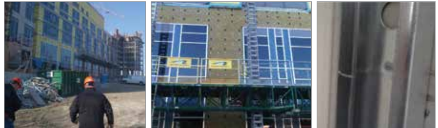
Exterior walls - Insulation to steel stud
