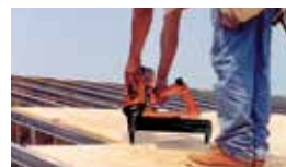
Plywood attachment—using TrakFast plywood to steel pin
