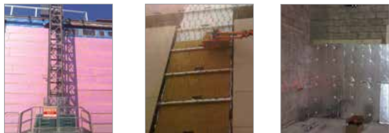
Exterior walls - Insulation to concrete
