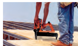
Plywood attachment—using TrakFast plywood to steel pin
