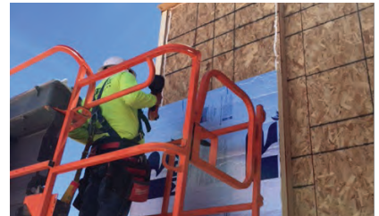
Behind cladding over wood stud walls
