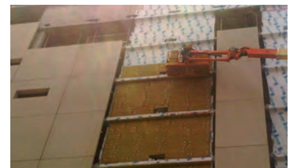
Behind cladding over concrete block walls
